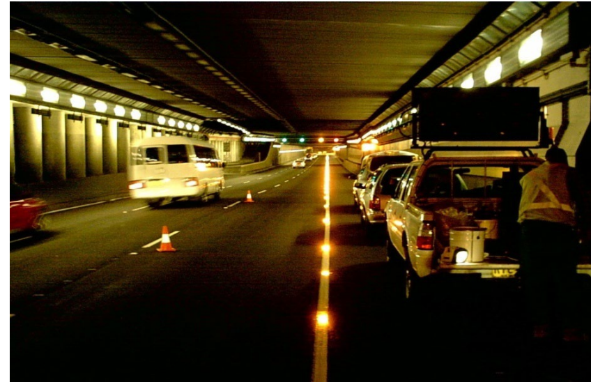
Tunnel (Sydney Australia)
