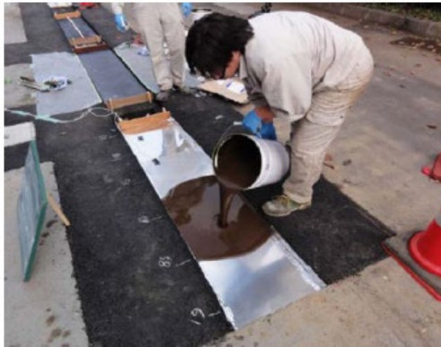
Figure14: Photograph showing the paving of the test road
